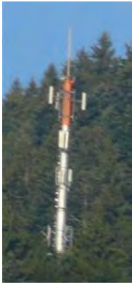
16 SEP 11: Ringberg mobile phone base station
