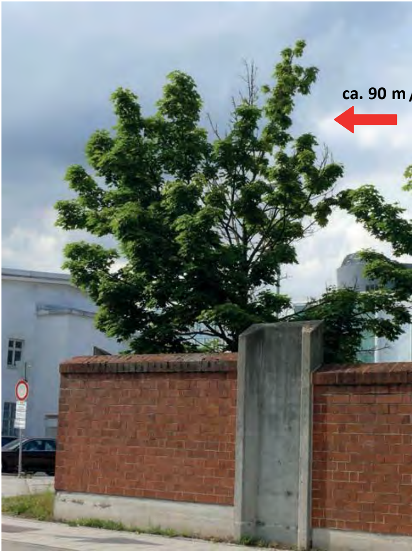
03 AUG 12: State Office for the Protection of the Constitution, southwest corner
