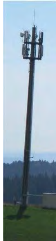
Mobile phone base station with 37 sector antennas and TETRA
