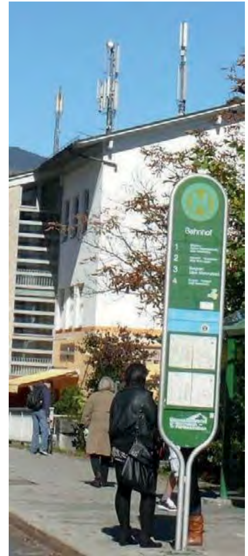
Mobile phone base station Bahnhofstraße
