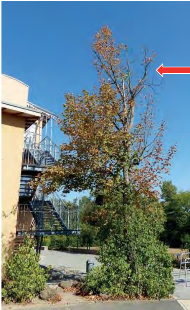
07 AUG 18: Ringastr., Waldorf school, sycamore tree (from SE), advanced damage, left and right side still show differences
